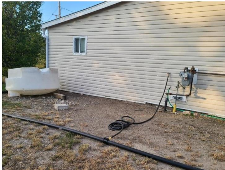
Temporary piping should not block any lanes, driveways or streets throughout the duration of construction. Where required, temporary ramps constructed of granular material, timber or other suitable material will be constructed to provide access.
